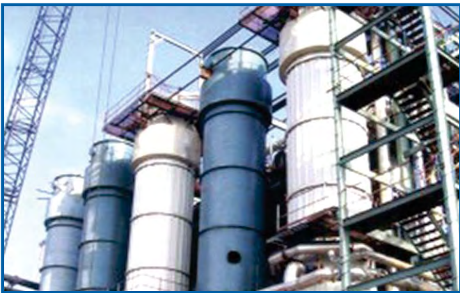
Falling Film Evaporator (Heating Surface 500m 2 to 6,000m 2 )
